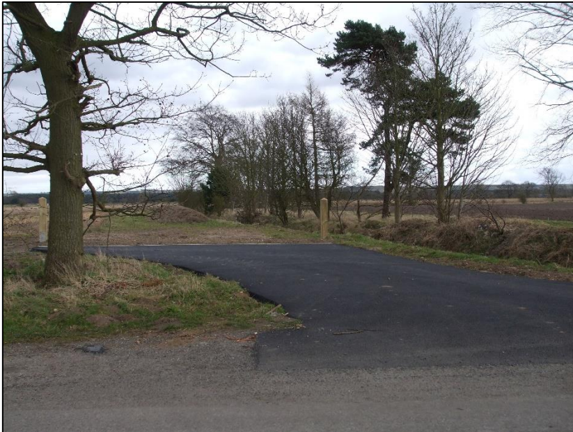
Photograph 1 Site Entrance as constructed 2018
